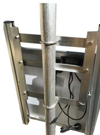
3. **Mark the mounting pole. This is where the top U-bolt will be.**
