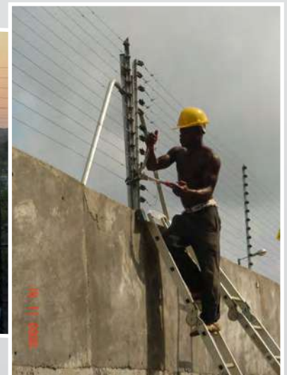
Petro Chemical Plant, Nigeria
