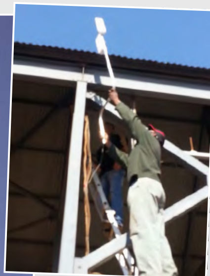
Wireless Repeater at Entrance
