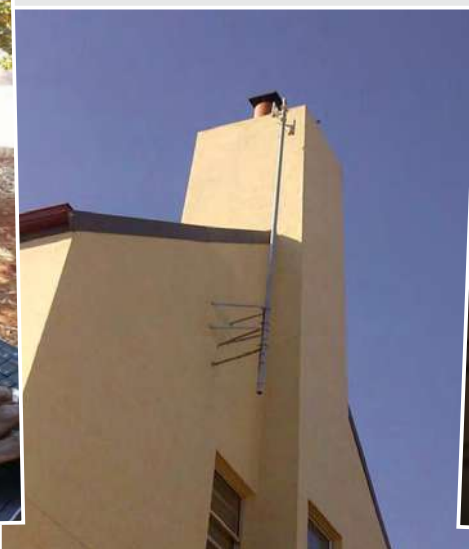
Wireless Antenna at Control Room
