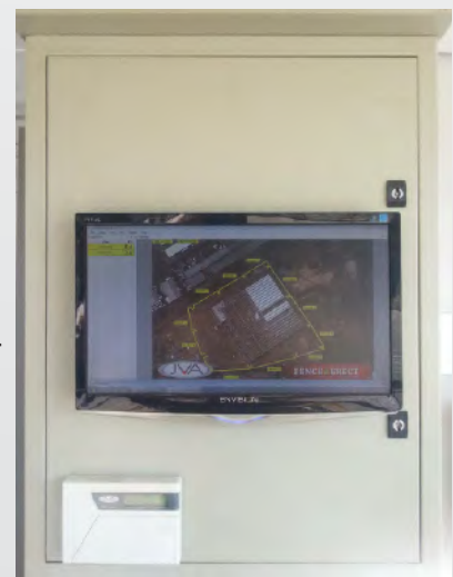
JVA ZM20 Mimic Installation
