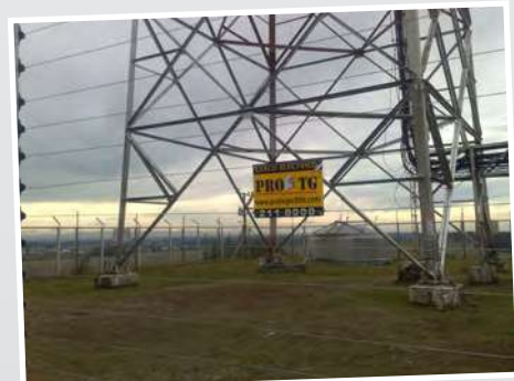
Power Station, Chili
