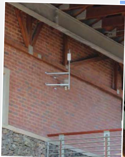
Wireless Antenna Installation
