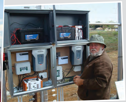
JVA security installation, Africa
