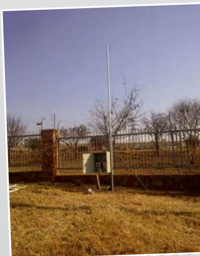
Wireless Repeater Station
