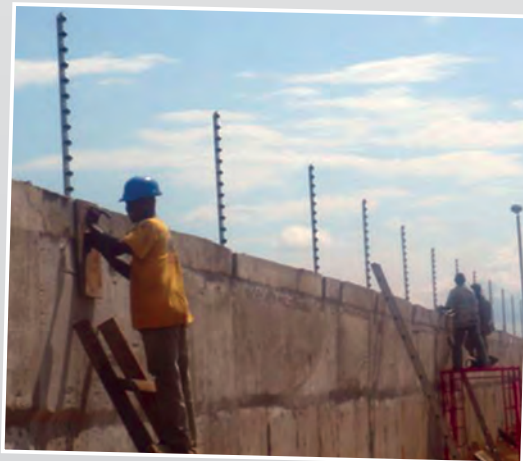
Security fence installation, India
