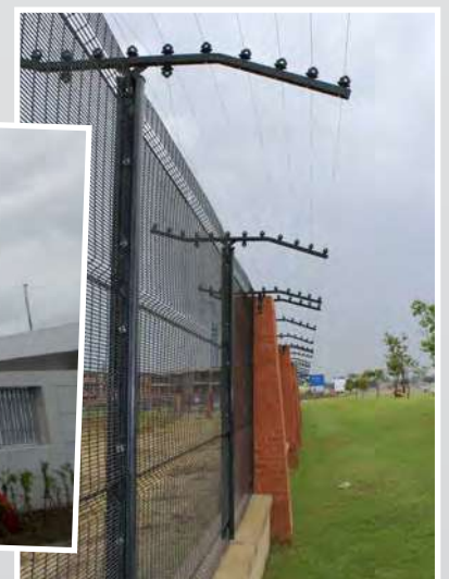
Estate Fence, Midrand (SA)
