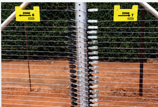
Synchronized System - Fence Line
