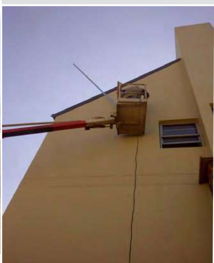
Wireless Antenna Installation
